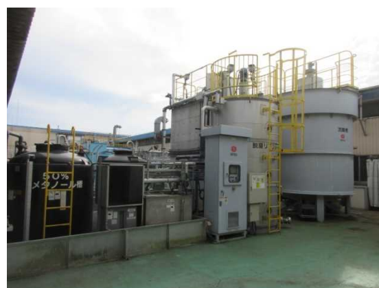
Moka Plant: biological denitrification wastewater treatment
