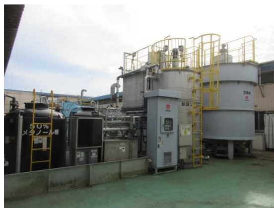
Moka Plant: biological denitrification wastewater treatment
