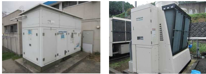
High-efficiency motor, inverter control compressor, cooling chiller
