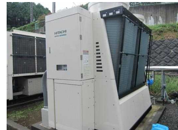
High-efficiency motor, inverter control compressor, cooling chiller
