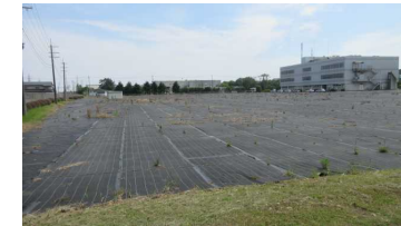
Site for the new Moka Plant
